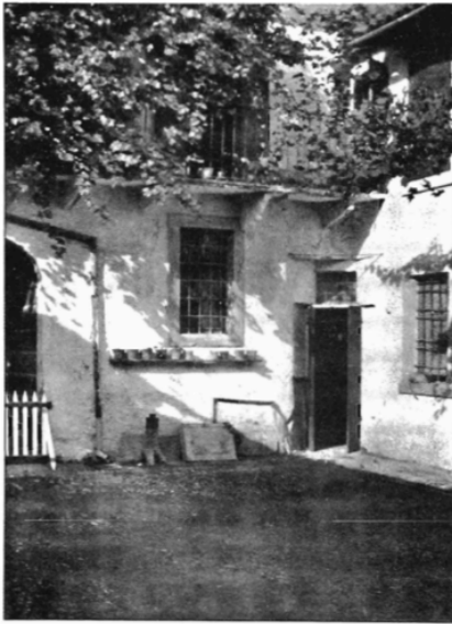
105 SOUTH FACING OUTDOORS**
